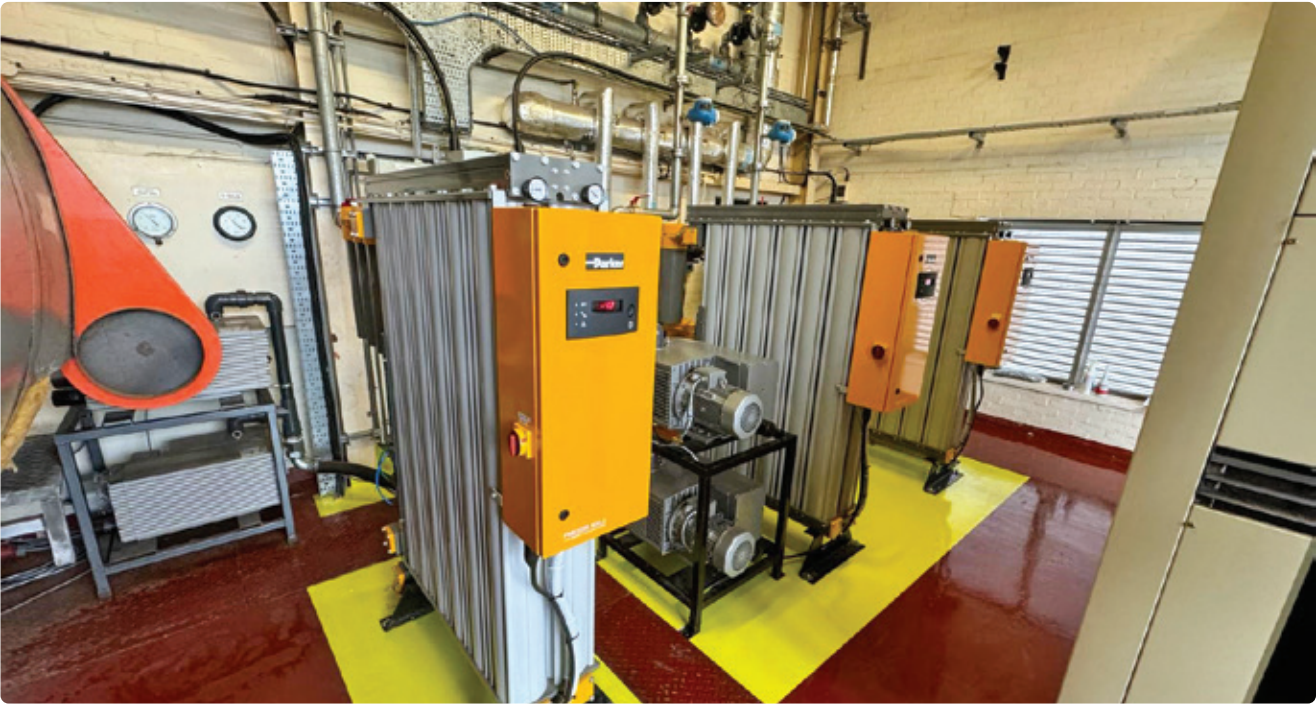
New compressed air dryer at Morpeth, UK
